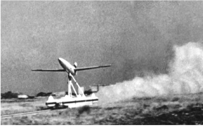
Above: Barnes Wallis's 'Wild Goose', an (intermittently) radio controlled model of his proposed supersonic 'aerodyne', thunders down the track on its rocket-propelled sled.
